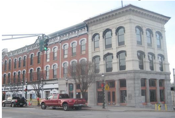
Figure 6.2: Renovated T.B. Flats Building, 12/2009
